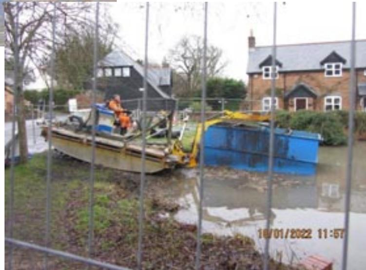
The work is being carried out by Hampshire County Council "Operation Resilience" and will take about two weeks. It involves removing the contaminated silt using a digger mounted on a floating pontoon. The silt is then emptied into the blue tank allowing the water to drain back into the pond. The silt is then removed by tanker and taken to an approved waste disposal site.
